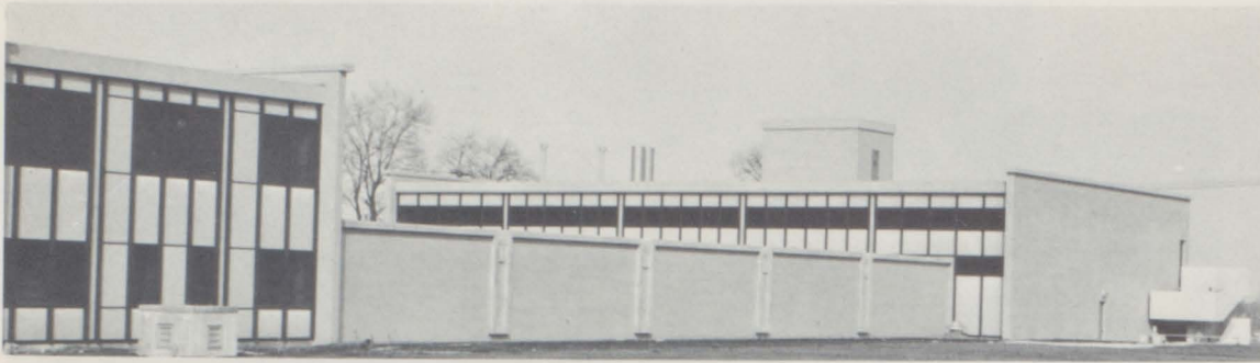
The water filtration plant, another symbol of modernization, provides pure, filtered water.
